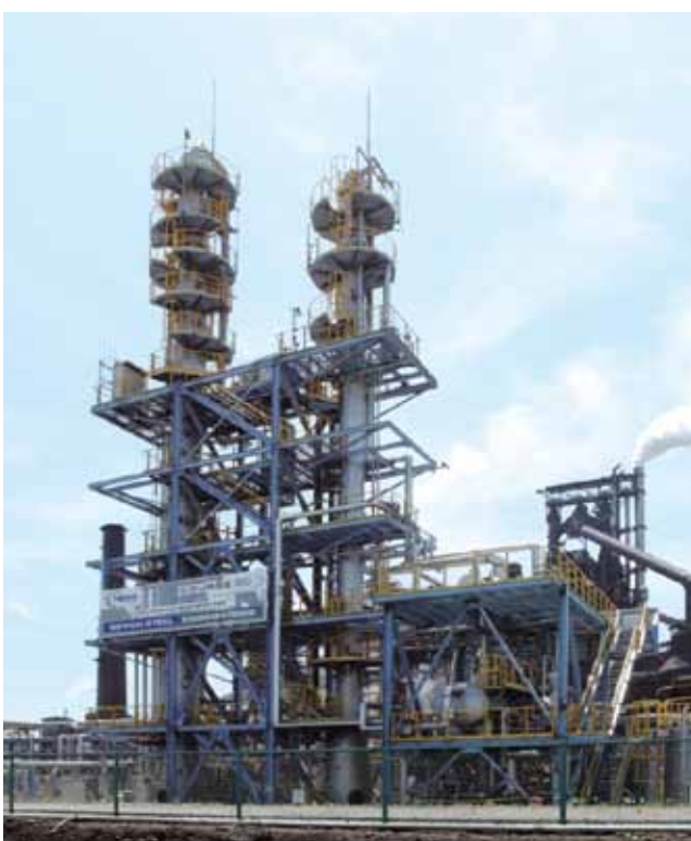
COURSE50 pilot plant for separating and capturing CO 2 [CAT-30]
